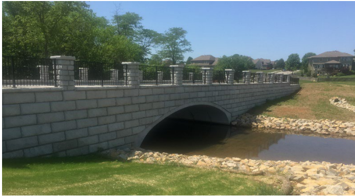
MSE large block headwall
