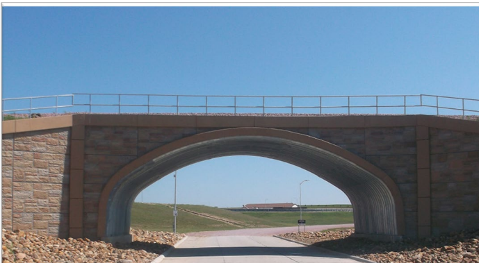
MSE Panel wall
