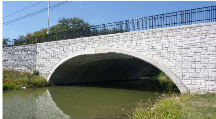
Concrete headwall w/ formliner
