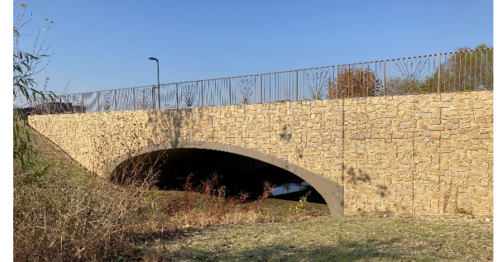
Precast headwall w/ formliner
