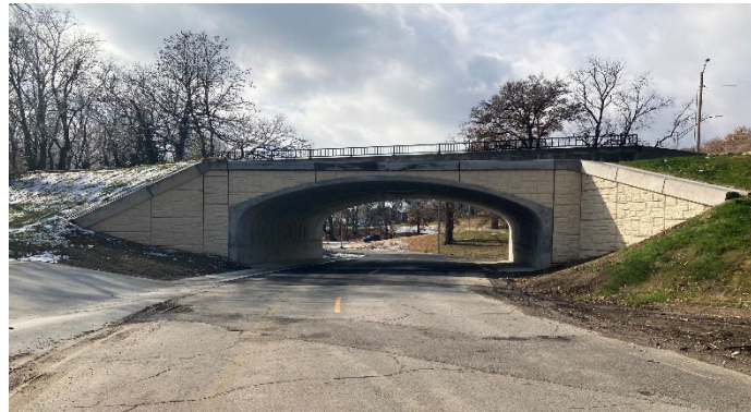
MSE panel wall
