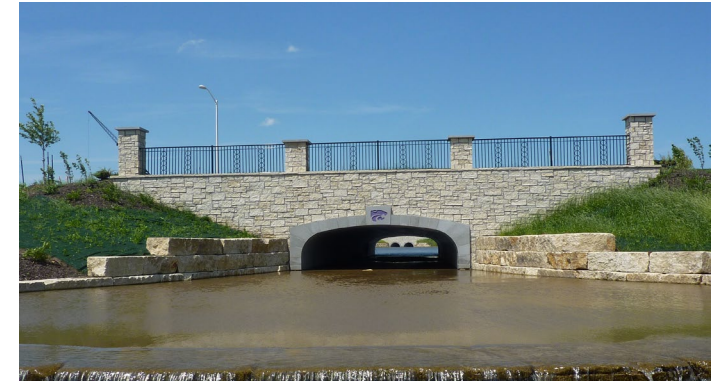
Concrete headwall w/ rock face
