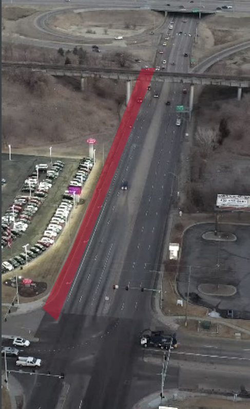
Right-side Ramp to Intersection
