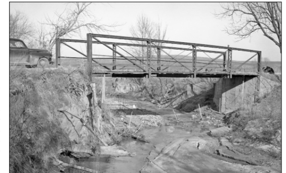
Photo: Bedstead truss Source: MoDOT
