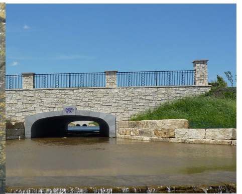
Headwall w/ rock face
