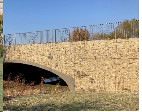
Headwall w/ formliner
