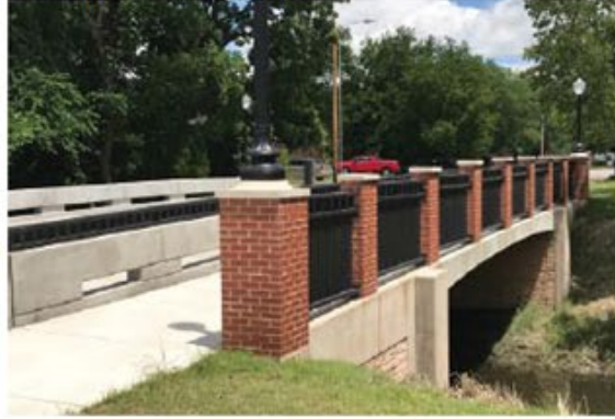
Decorative Columns / Lighting
