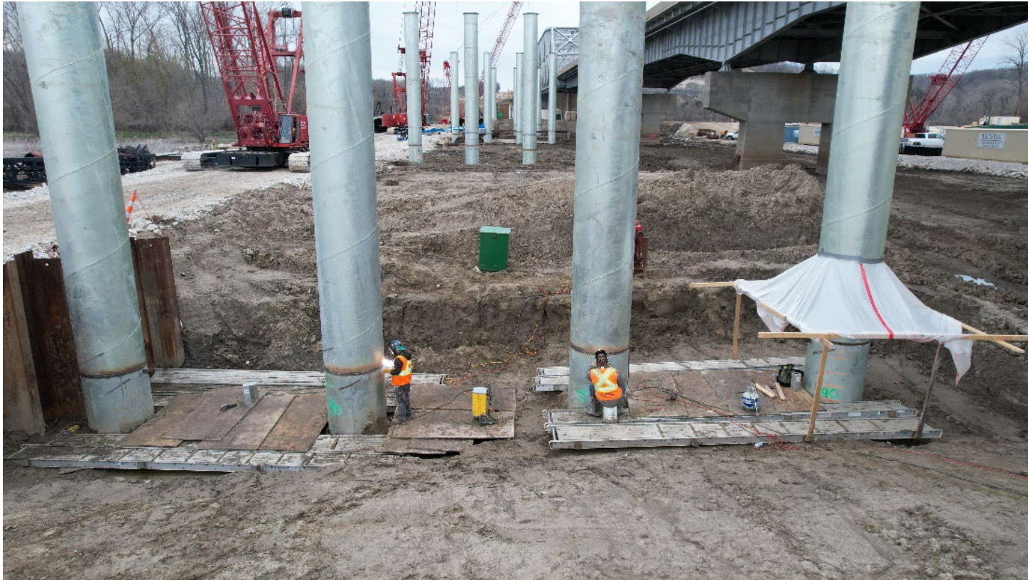
Welding 48" Galvanized Pipe Piles
