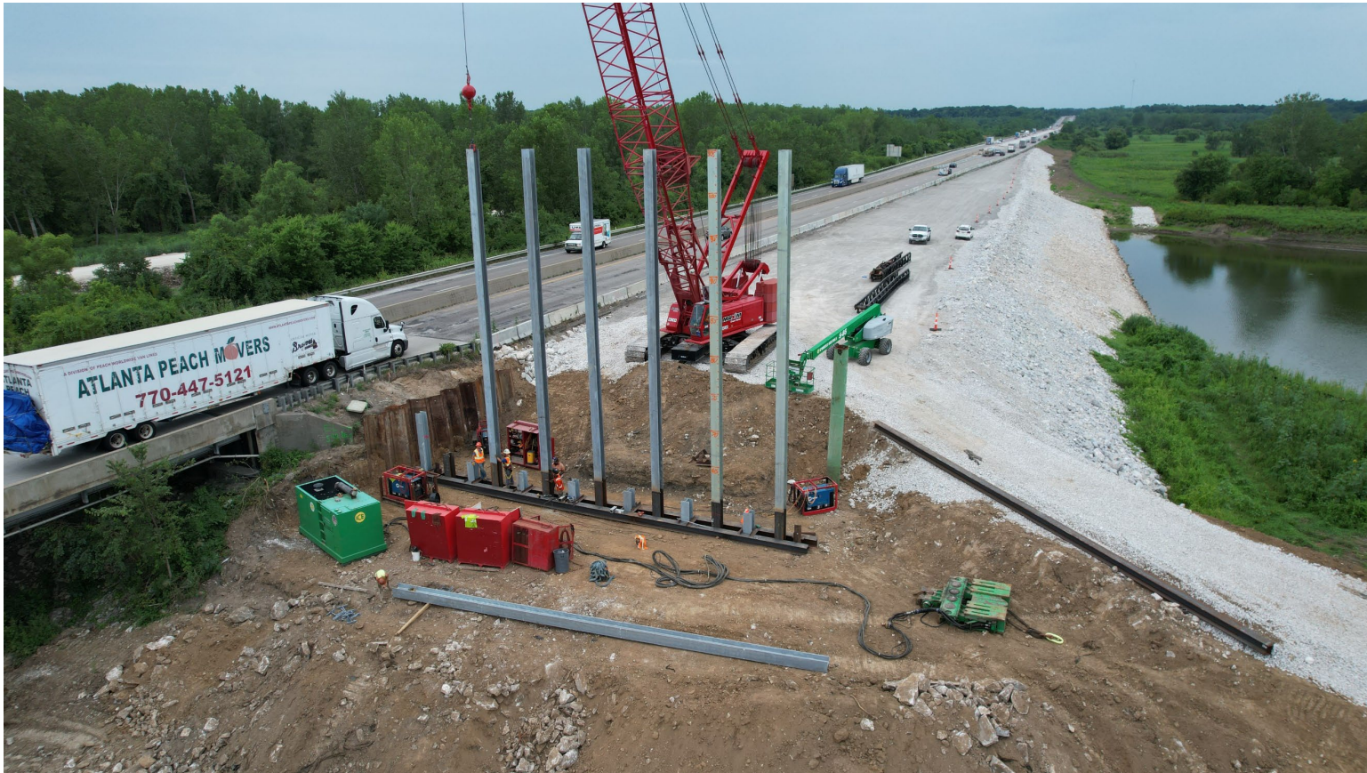
West Abutment H-piles
