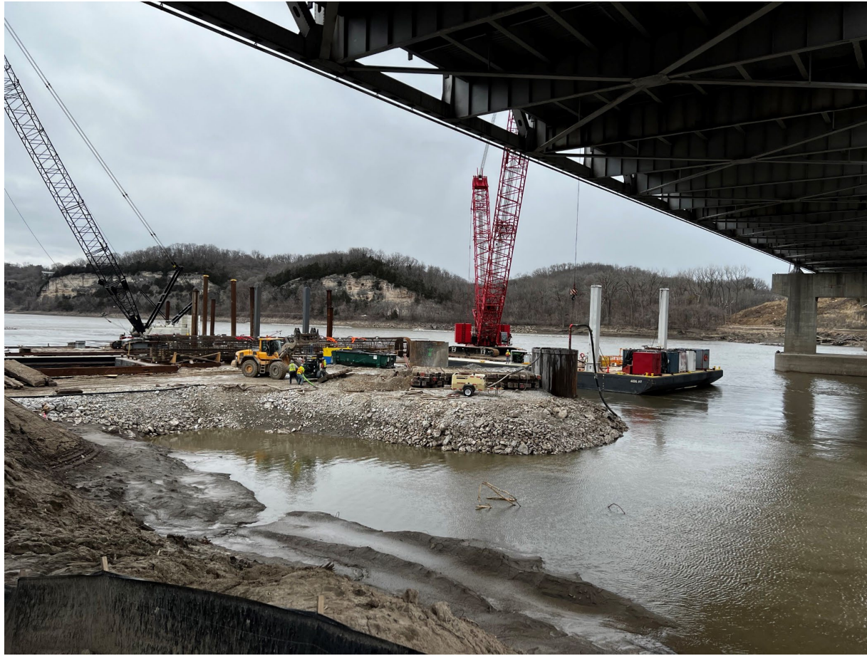
Drilling Shafts at Bent 12
