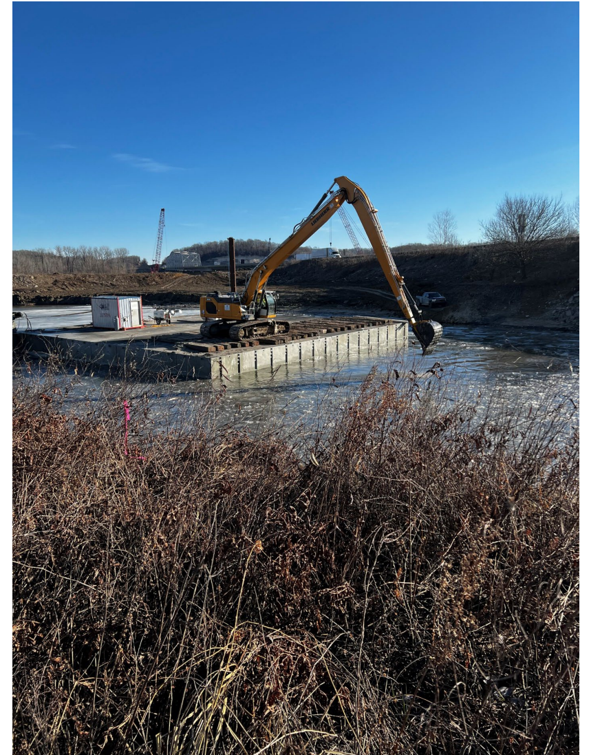
Muck Removal for Embankment
