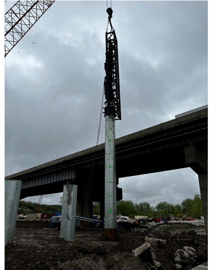
Driving Pipe Pile
