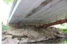
Underside Southeast Quadrant
