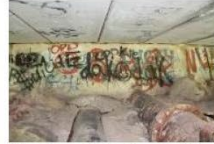
Drainage Culvert and Sanitary Sewer at South Abutment
