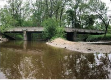
HNTB, Bridge Scoping Report
