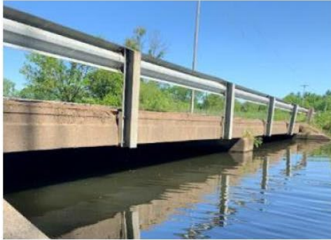
HNTB, Bridge Scoping Report
