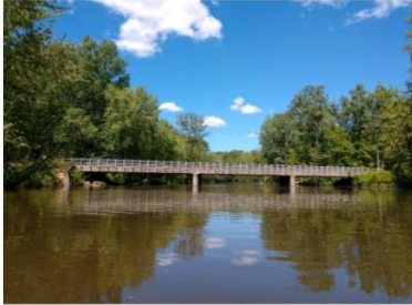
HNTB, Bridge Scoping Report
