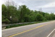
SE Guardrail and Overhead Utilities
