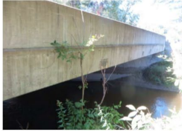
HNTB, Bridge Scoping Report
