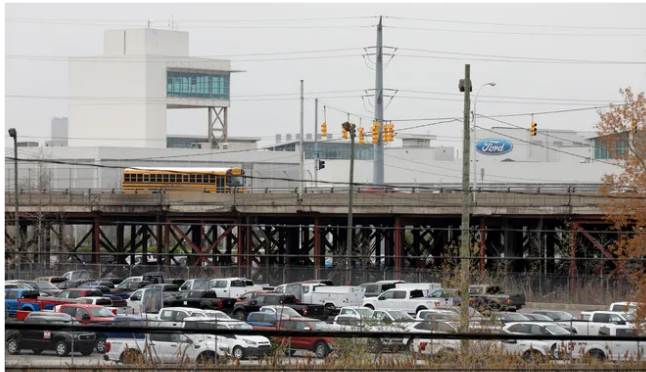
A school bus and other vehicles cross over the Miller Road Bridge in Dearborn with part of the Ford Motor Company Dearborn Truck Plant in the background on Thursday, April 2, 2019. Eric Seals, Detroit Free Press
