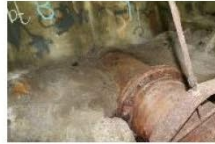
Sanitary Sewer at North Abutment
