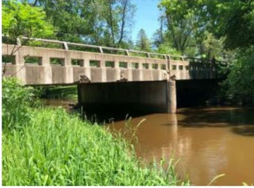
HNTB, Bridge Scoping Report
