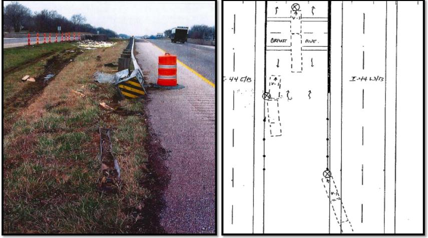
Truck was traveling westbound on I-44, drifted off the roadway, struck the guardrail, got behind the guardrail, collided with the inside eastbound bridge rail, became airborne and landed on Grant street under the I-44 overpass.
