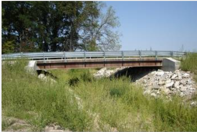
Audrain County, MO Bridge 411 Built 2012 Steel 4 Girders 47.5 ft. Span 24 ft. Roadway Width 2 ft. Structural Depth No Skew
