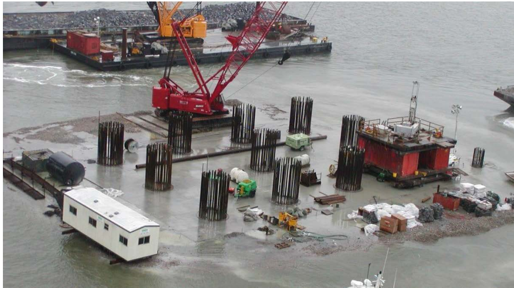
West Tower Drilled Shaft Foundations Arthur Ravenel Jr. Bridge, Charleston SC
